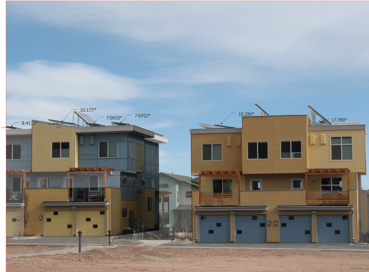
Figure C.1: Solar array angles measured using Google Sketchup [4] with a 3D axis aligned to the building. The duplex units have a slightly higher solar array angle than the 5-plex units with the exception of the 5-plex array mounted on the sloped roof.
