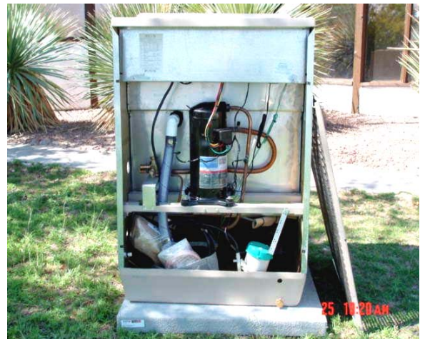
The FREUS Condenser Must Be Level, To Insure Proper Water Distribution Over The Condenser Coil
