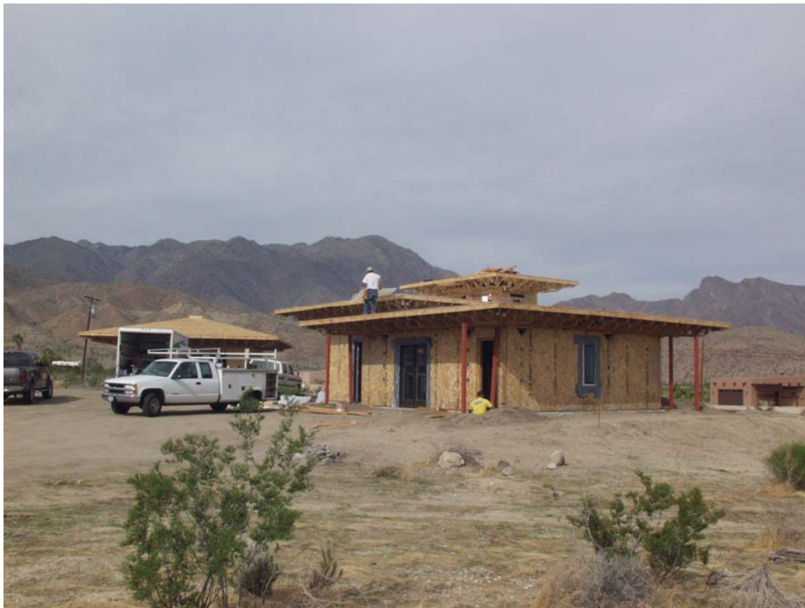
Figure 3 Broken Arrow Prototype Under Construction
