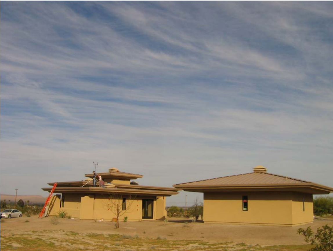
Figure 7 East Star Prototype Completed
