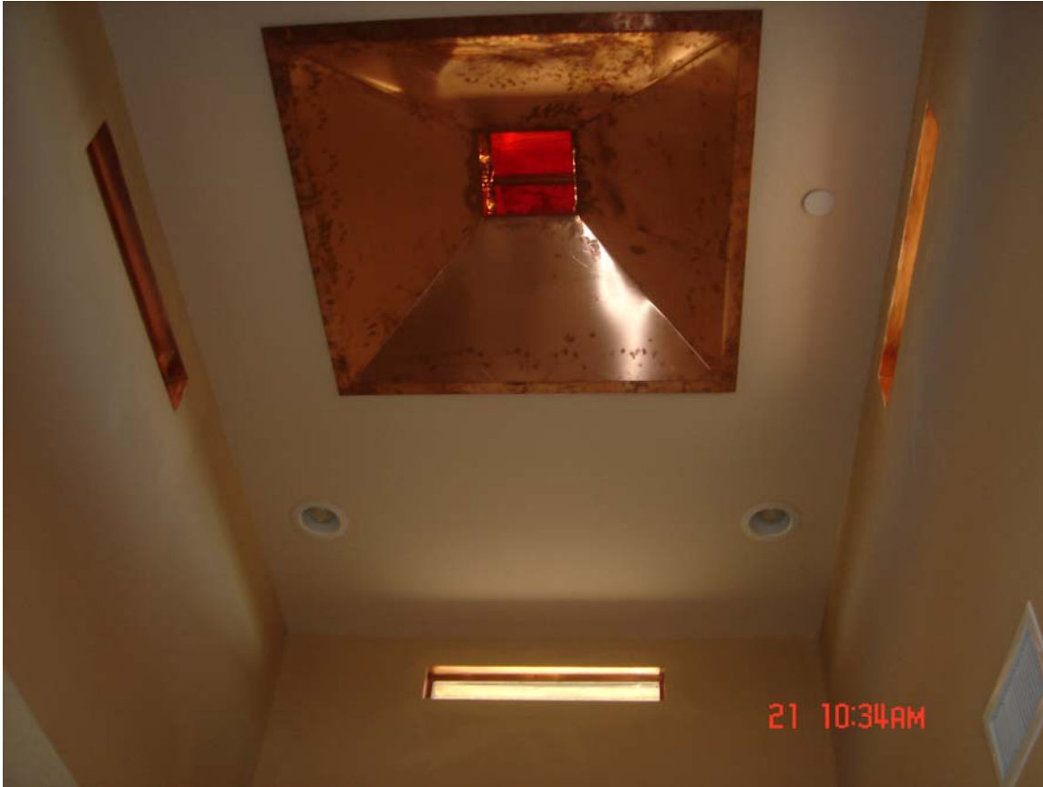
Figure 9 Copper Flashed Skylight Typical of Borrego Prototypes
